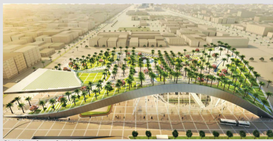
Olaya Metro Station, Saudi Arabia
